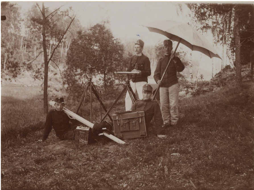
Figure 2: Surveying team in France, 1908, using theodolites for fixing a control point and plane tables for recording topography and parcel boundaries.
